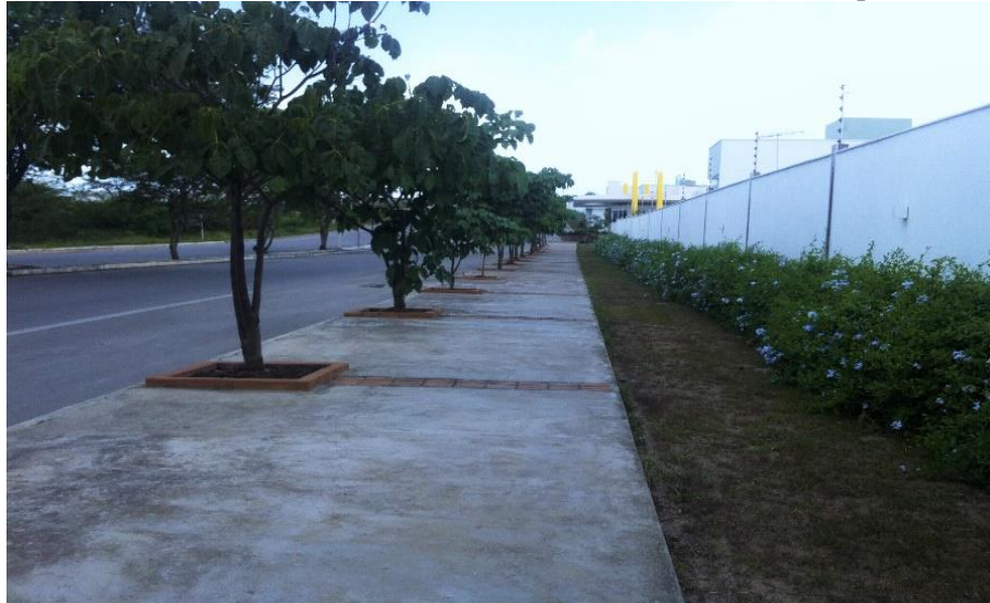
Figura 2 – Muro frontal do condomínio Serraville Residence Privê, Campina Grande (PB)
